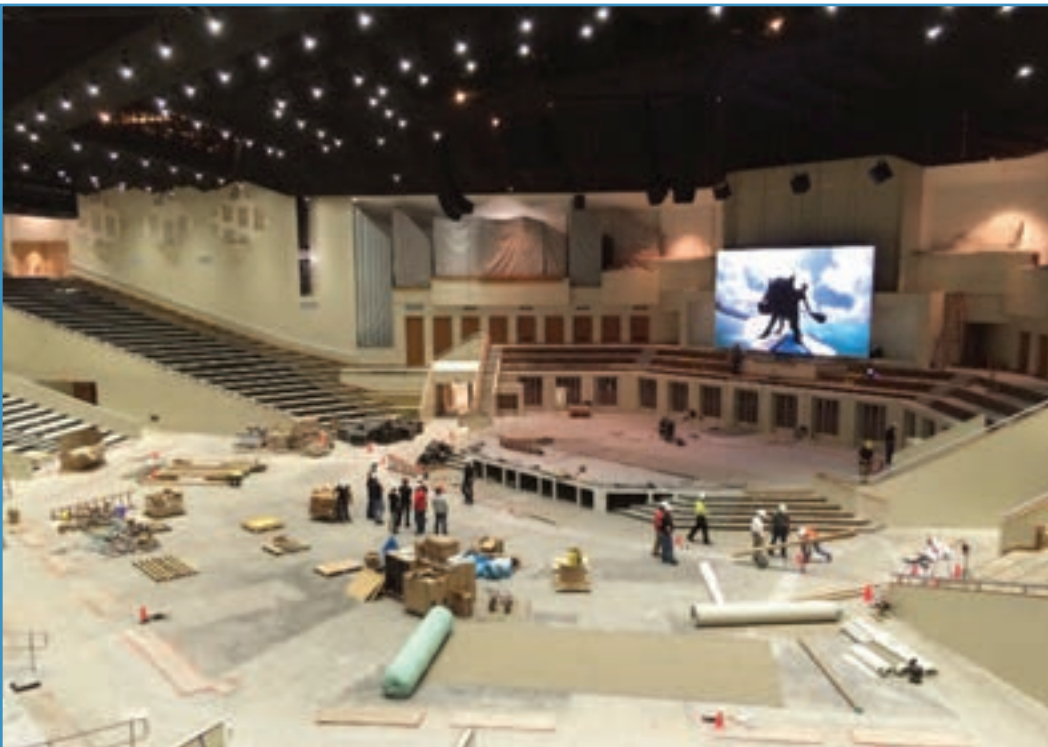
During renovations, the auditorium was stripped to its concrete foundation. Above: The Vanguard LED screen has been assembled and is undergoing testing prior to being hung in its final position.
