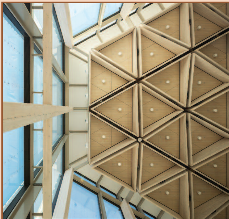
A motif embedded in the original construction, the hexagon shape is repeated in virtually every part of the building. Here, the wood triangulation visible in the ceiling is the roof structure. Prefabricated Douglas fir triangulated glue-lam cofferes ganged in linear swaths up to 65' long were prefabricated off-site to save time.
