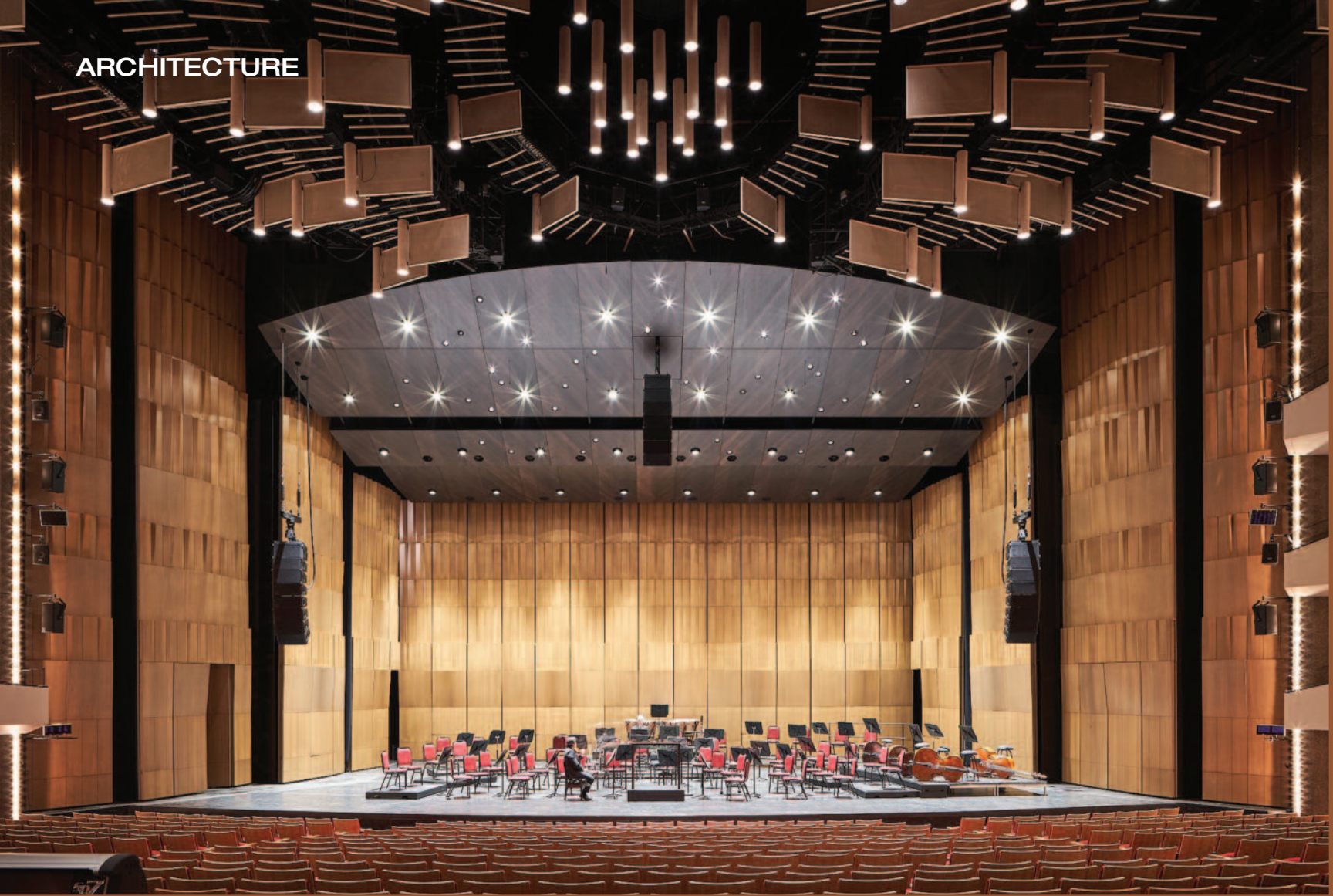
Southam Hall's new orchestra shell consists of an upstage wall, overhead forestage reflector, and five movable towers on each side of the stage, four of which are visible in the orchestra configuration. Finished on one side in white oak, the panels can be manually flipped and rearranged with their opposite dark sides toward the stage and audience for other types of performances.
