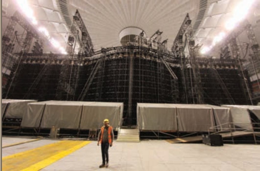
A different view of the curved screen, while the cantilevers are being built.
