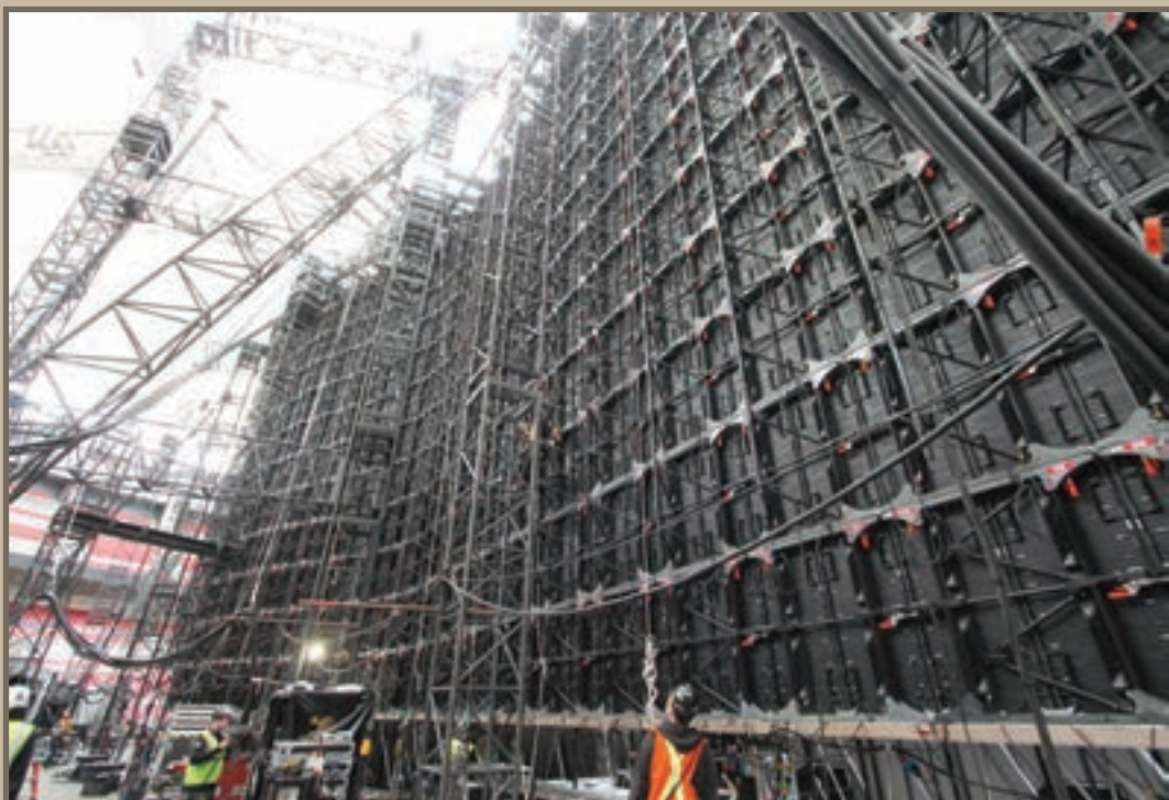
The back of the screen, with the SPACEFRAME wind bracing in place.
