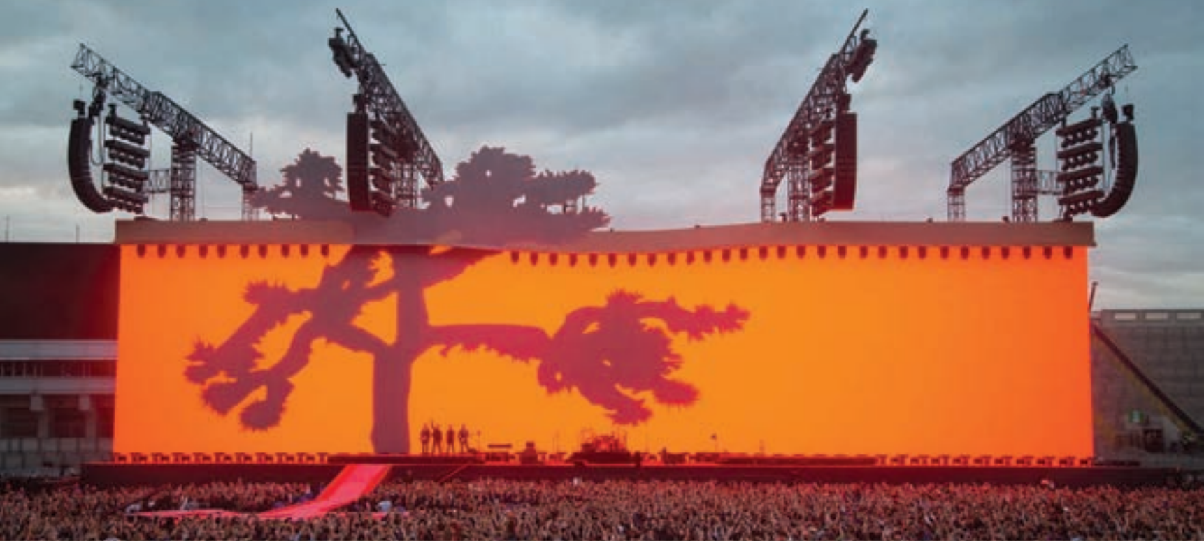
The cantilevers are used for the Clair Cohesion PA and also for lighting positions.
